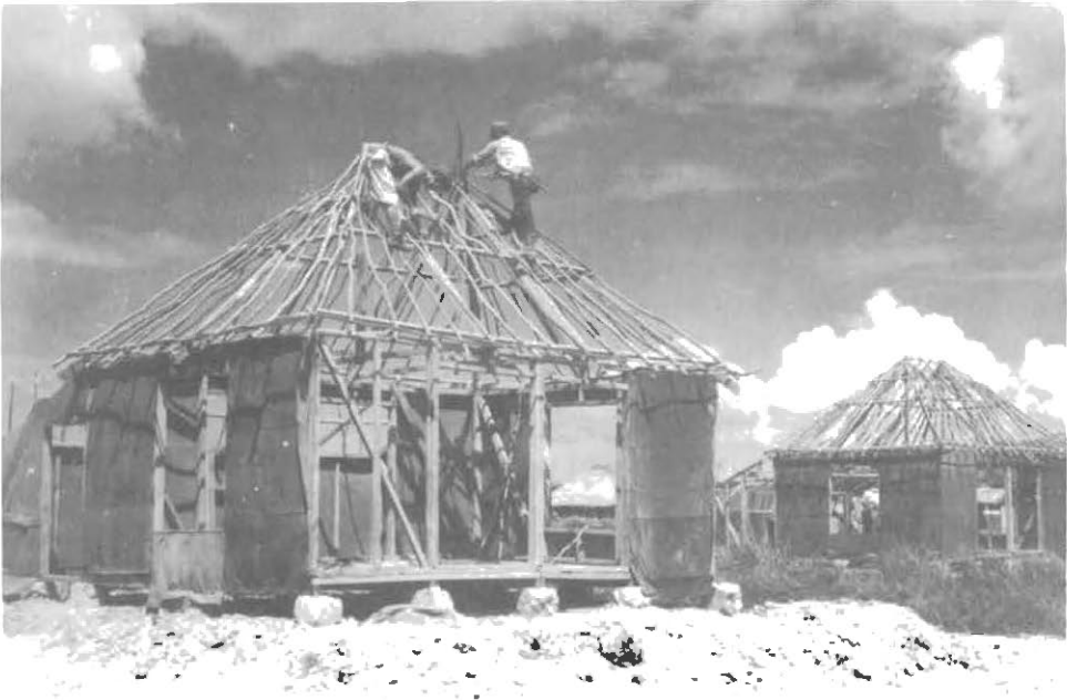
STANDARDIZED HOUSING being constructed under military government supervision.
