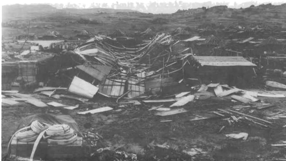
TYPHOON "LIBBY" destroyed this building on Okinawa in October 1948.
