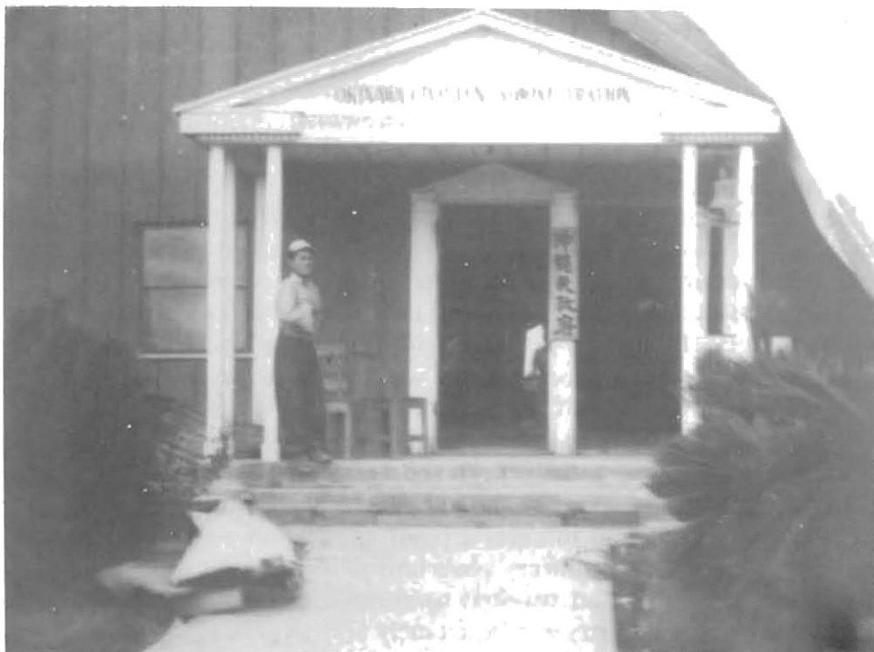
TYPHOON DAMAGE. Typhoon "Libby" destroyed the roof of this local government building in October 1948.
